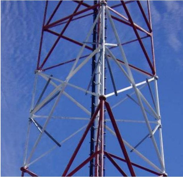
Fig. 11 Reinforcement of diagonal braces – shortening the buckling length in the plane of the tower wall
