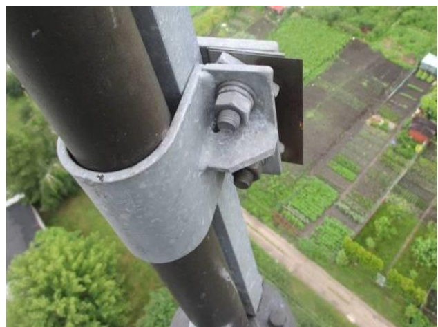
Fig. 12 Leg reinforcement – additional C-sections mounted by means of clamps
