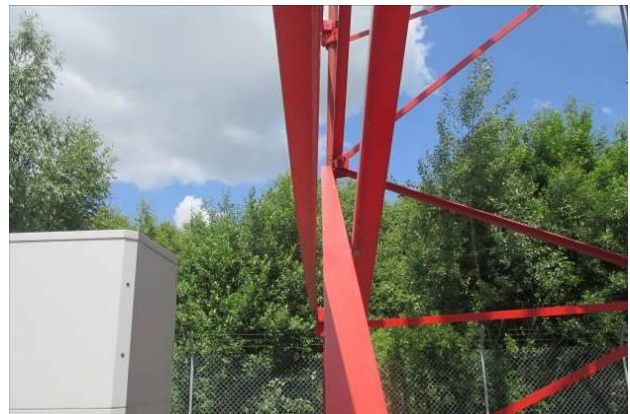
Fig. 4 Leg reinforcement – an additional horizontal bracing member with no connection at the node
