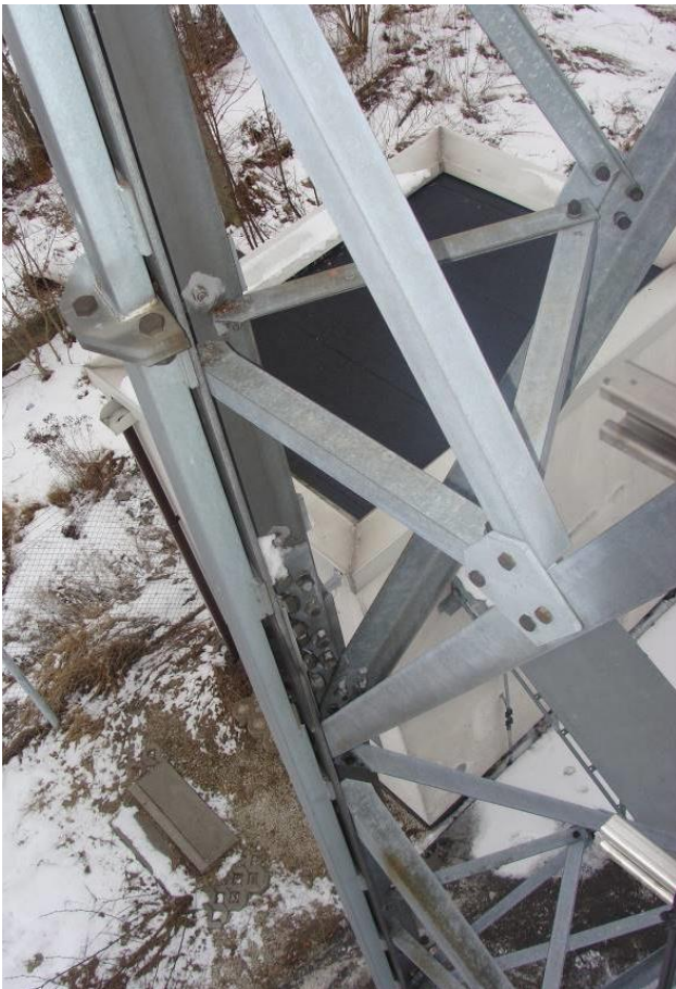
Fig. 13 Leg reinforcement – additional C-sections mounted by means of spacers
