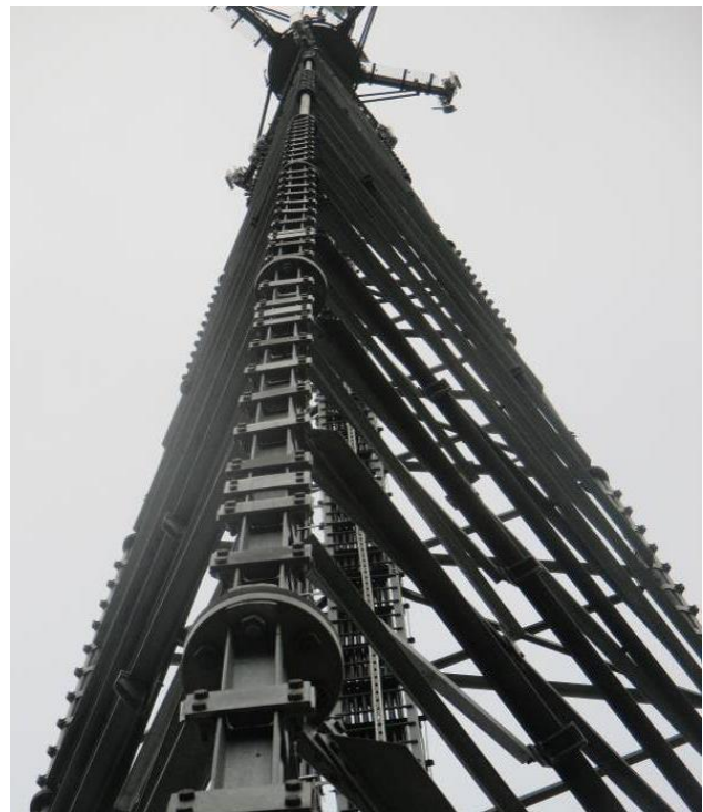
Fig. 11 Reinforcement of diagonal braces – shortening the buckling length in the plane of the tower wall
