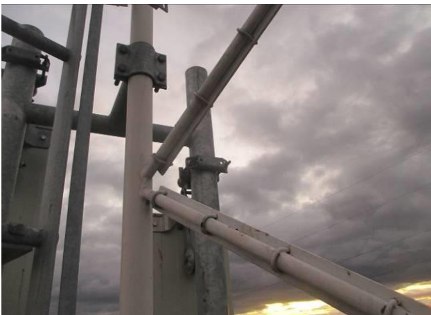
Fig. 15 Increasing the cross-section of diagonal braces by attaching additional flat bars and C-sections to existing members
