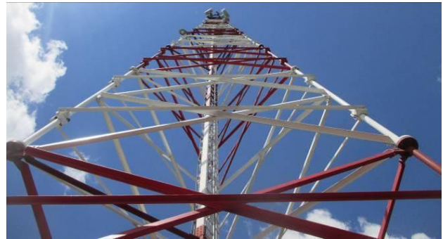
Fig. 1 Leg reinforcement – an additional horizontal bracing member fixed with one bolt
