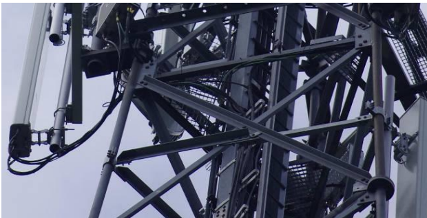
Fig. 3 Leg reinforcement – an additional horizontal bracing member joined below the node with a movable piece of sheet plate
