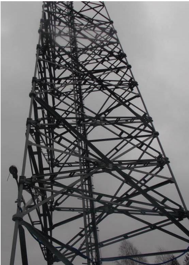
Fig. 5 Leg reinforcement – an additional X-bracing pattern made of framework members
