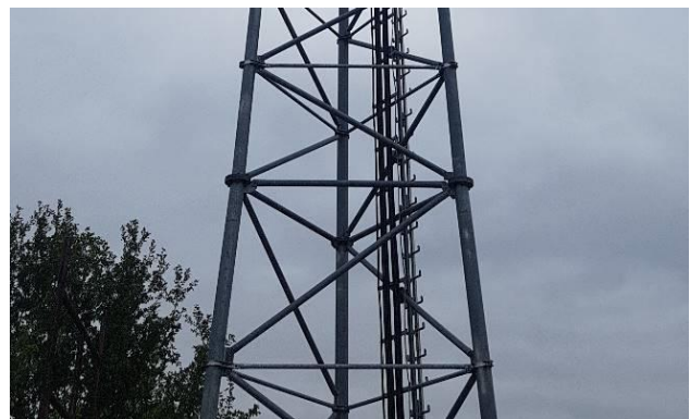
Fig. 9 Leg reinforcement in a tower with a single bracing pattern – additional cross-bars
