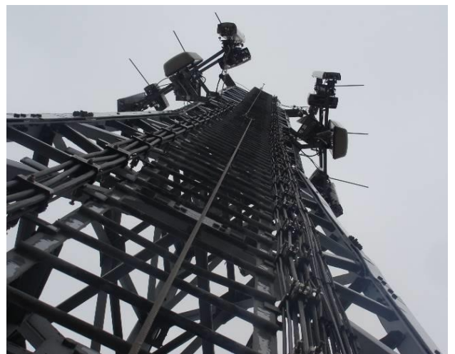
Fig. 14 Leg reinforcement – additional members in the form of flat bars, not integrated with the existing structure
