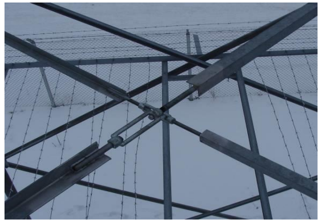
Fig. 16 Stiffening a tower structure in the form of horizontal diaphragms to prevent its twist
