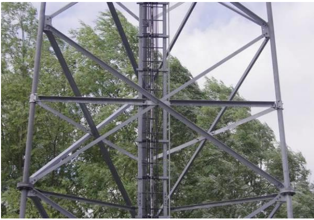
Fig. 1 Leg reinforcement – an additional horizontal bracing member fixed with one bolt
